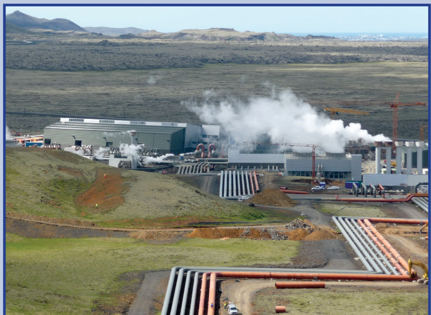
Geo-thermal Power Plant at Hellisheidi, Iceland
