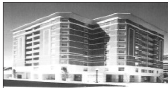
High-rise Apartment Building in Arlington, Virginia; Sold earlier this year
